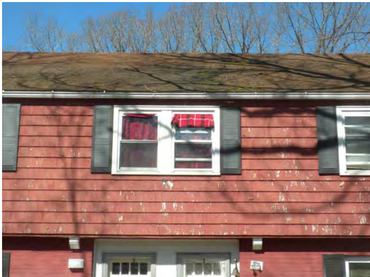
Peeling paint was observed with respect to most wood shake siding
