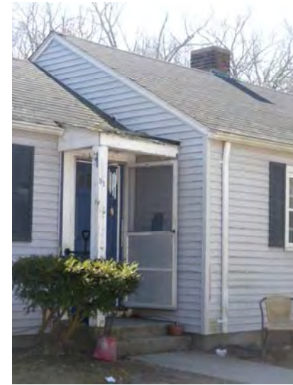
Painted wood canopies at the doorways of A type buildings exhibit wood rot and peeling paint.
